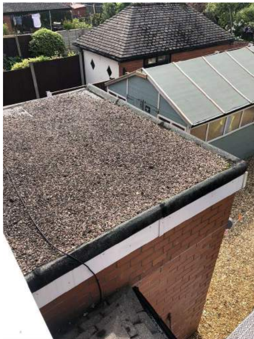
Flat rear extension roof.
