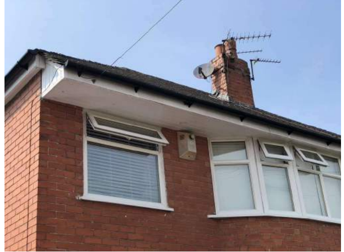
Front gutter and fascia and soffit.
