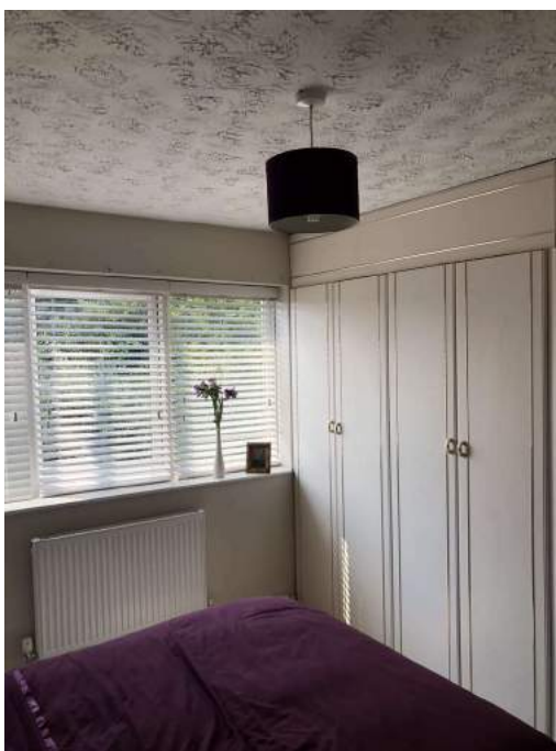
Radiator and TRV.
