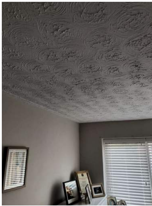
Textured ceiling in rear bedroom.
