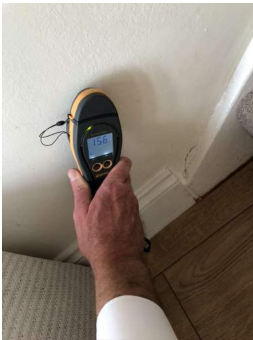
Internal wall damp check.
