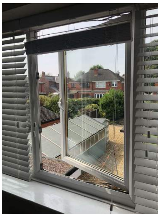
Rear fire escape window.
