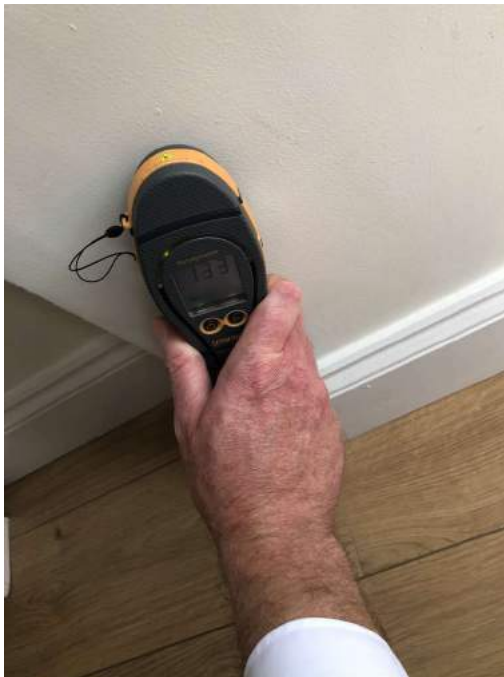
Internal wall damp meter check.
