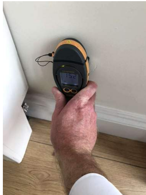
Internal wall damp meter check.
