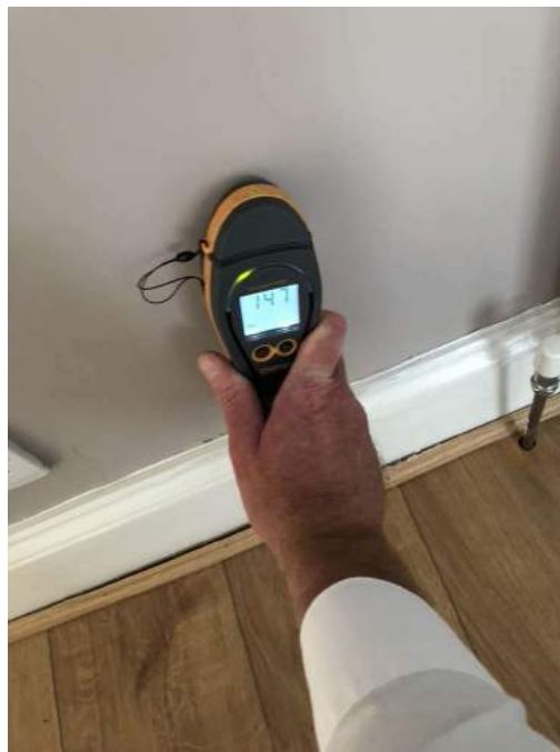
Internal wall damp check.
