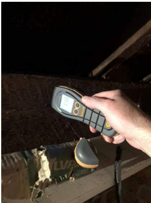
Purlin damp check.
