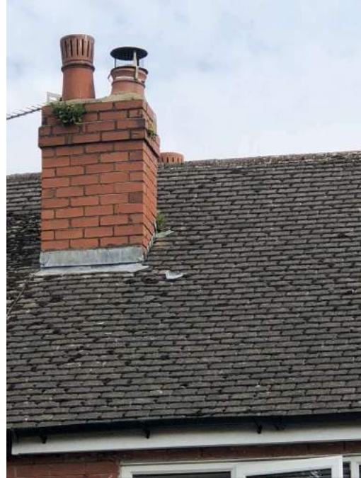
Rear chimney stack.
