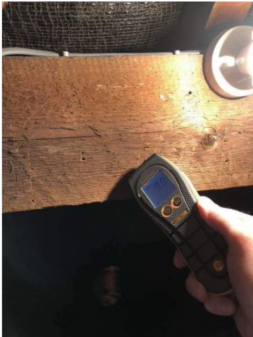
Purlin damp check.
