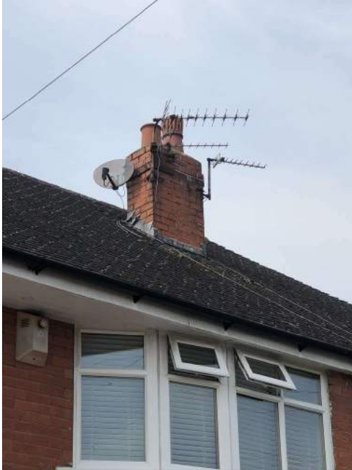
Front chimney stack.
