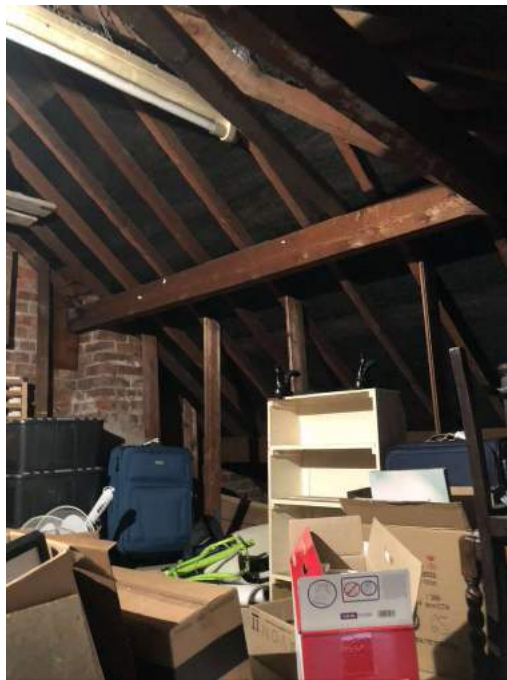
Rafters, purlin and hangers.
