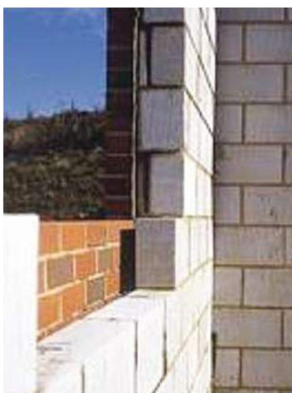
Modern cavity walls under construction
