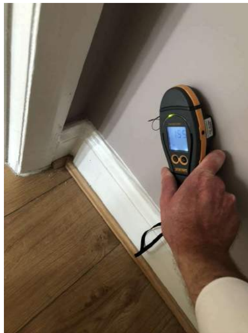
Internal wall damp check.
