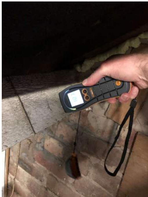
Purlin damp check.
