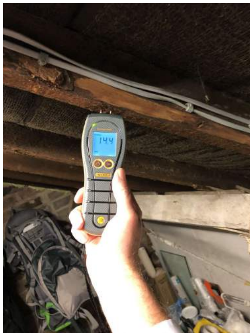
Rafter damp check.
