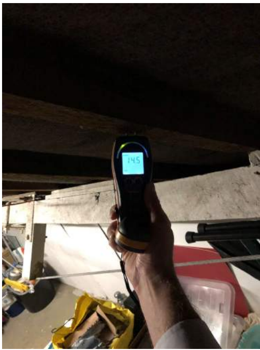
Rafter damp check.
