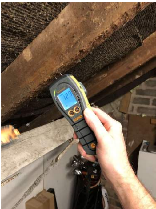
Rafter damp check.
