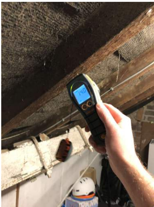
Rafter damp check.
