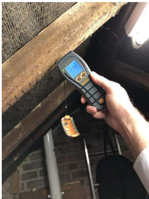
Rafter damp check.
