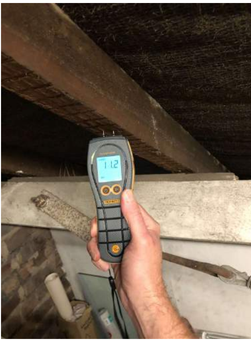
Rafter damp check.
