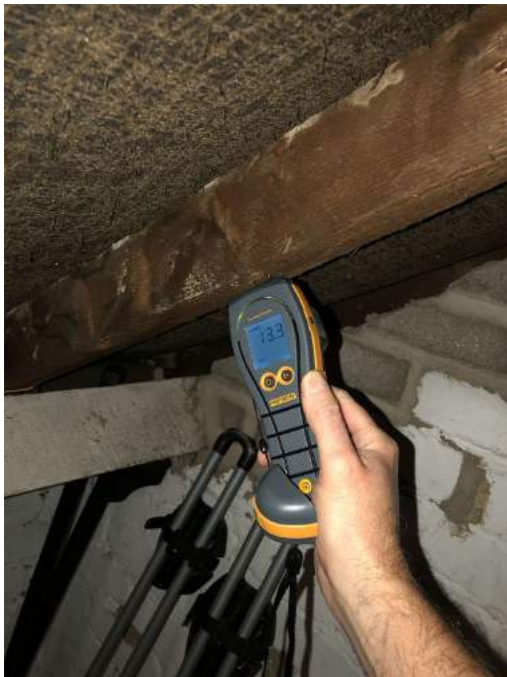
Rafter damp check.
