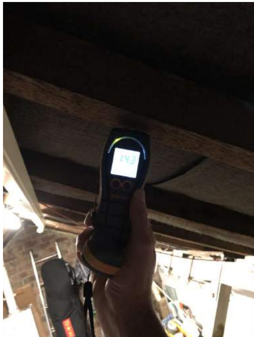
Rafter damp check.
