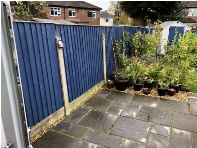
Boundary fence and posts.
