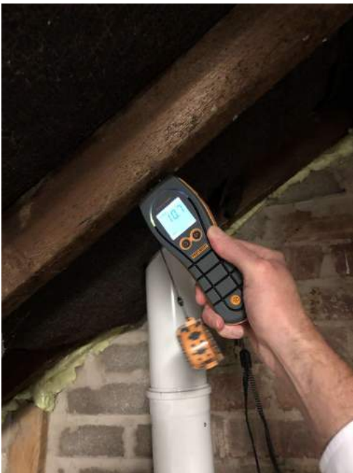
Rafter damp check.
