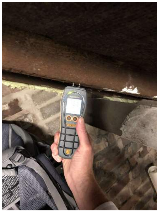
Rafter damp check.
