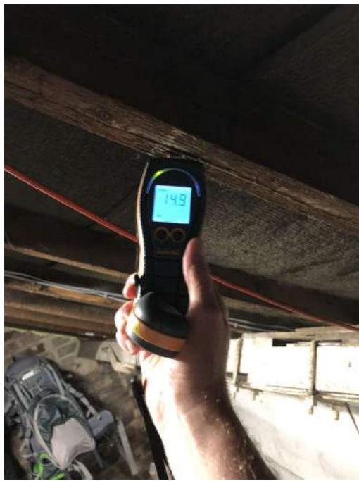
Rafter damp check.
