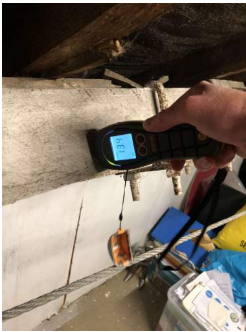
Purlin damp check.
