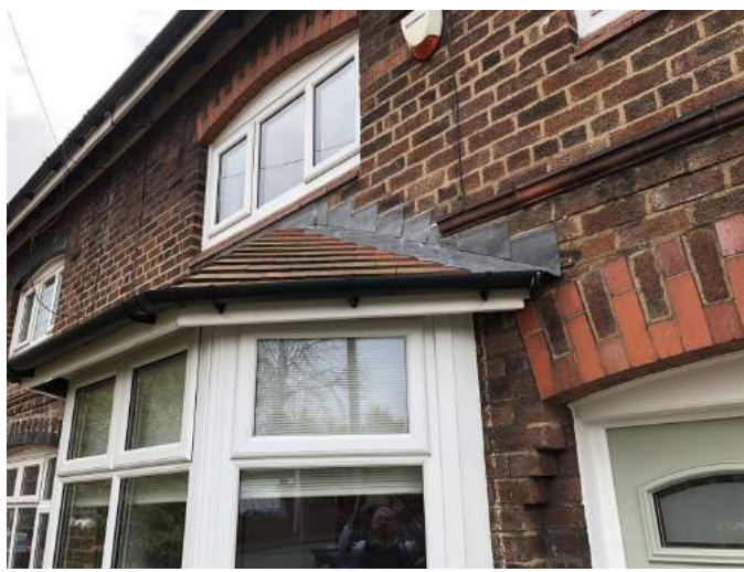
Front bay window lead flashing.
