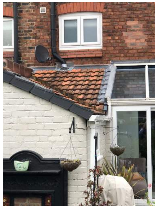
Rear roof and lead flashing.
