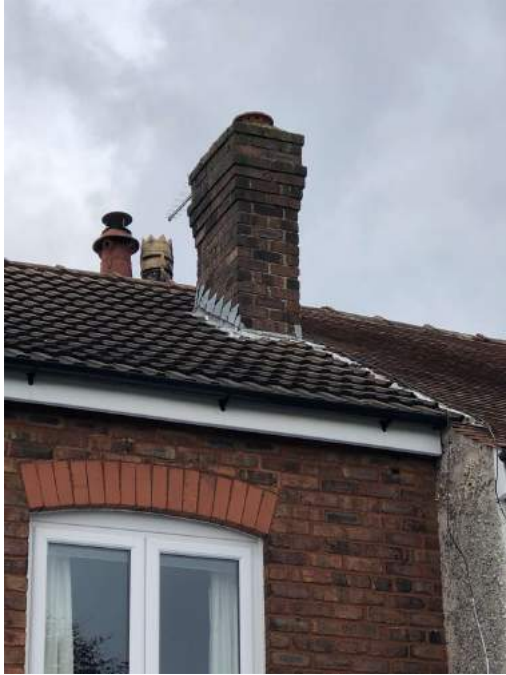
Rear chimney stack.
