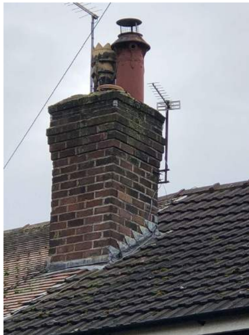
Front chimney stack, flues and lead flashing.
