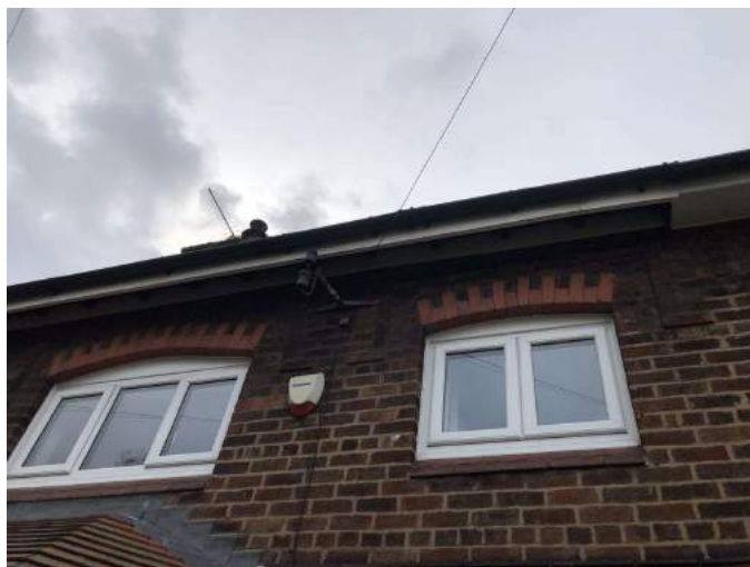
UPVC gutter and fascia.
