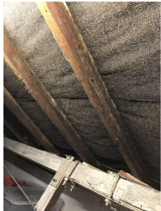
Rafters and sarking felt.
