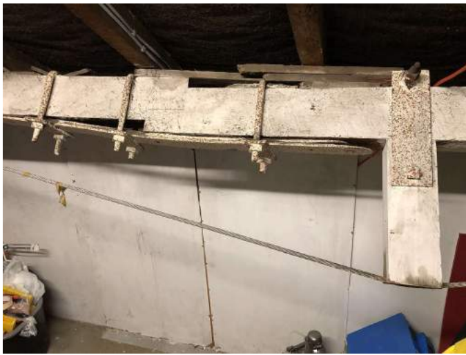
Purlin brackets and packers.
