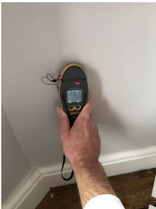
Internal damp check. High reading.
