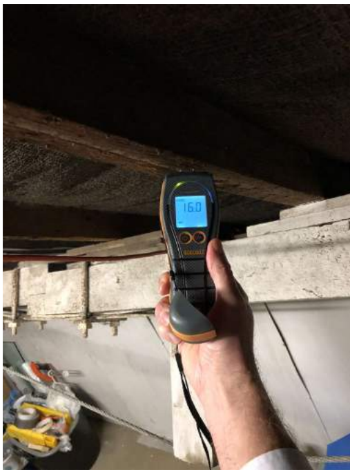
Rafter damp check.
