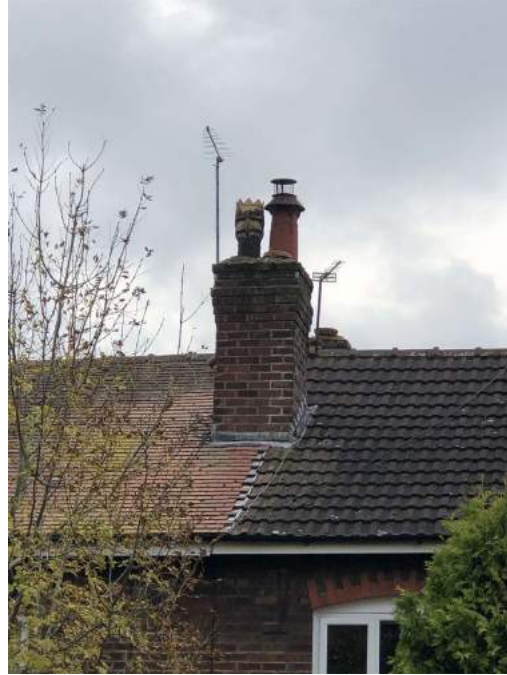
Front chimney stack.
