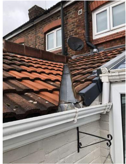
Rear roof and valley.
