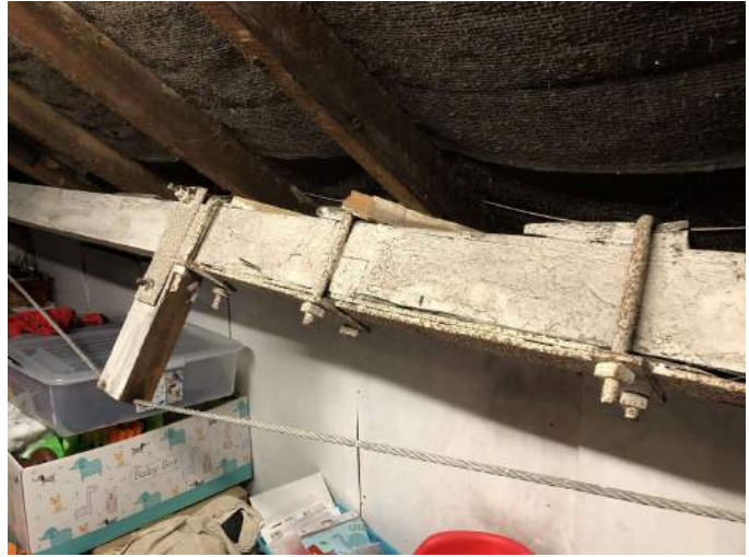
Purlin, brackets and packers.
