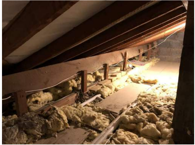
Purlin, hangers and rafters.
