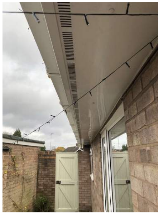
Gutter and soffit.
