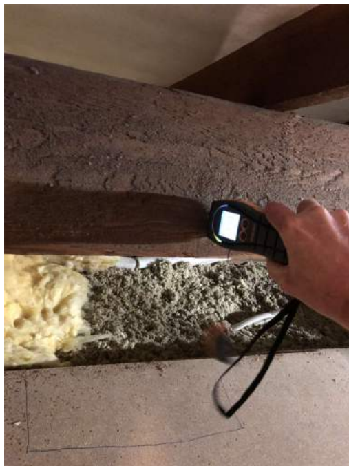
Purlin damp check.
