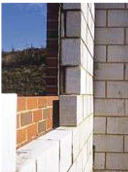
Modern cavity walls under construction
