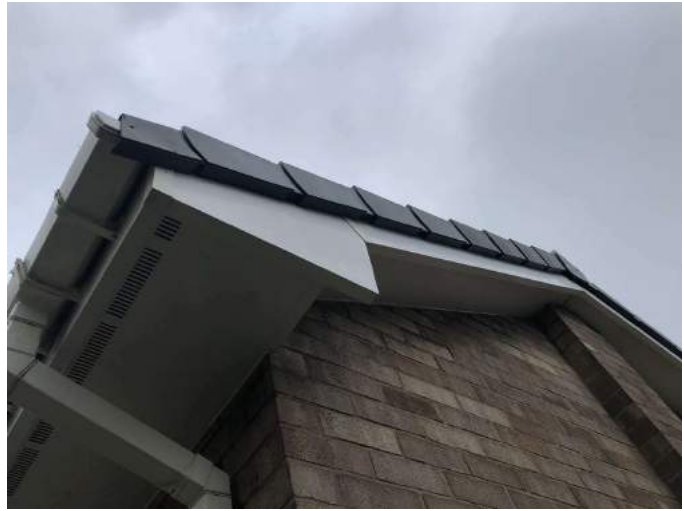
Dry verge covers, fascia and soffit.
