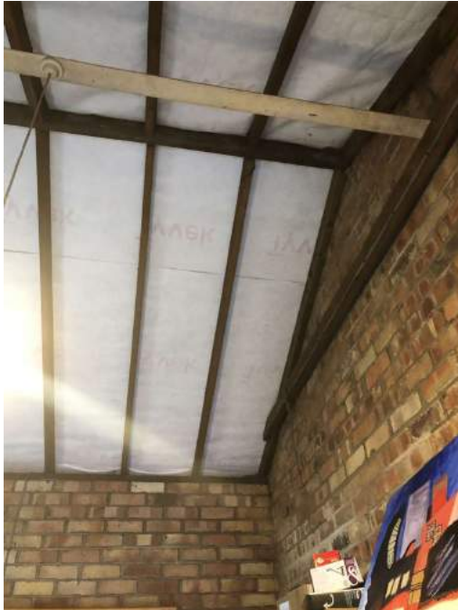
Garage roof construction.
