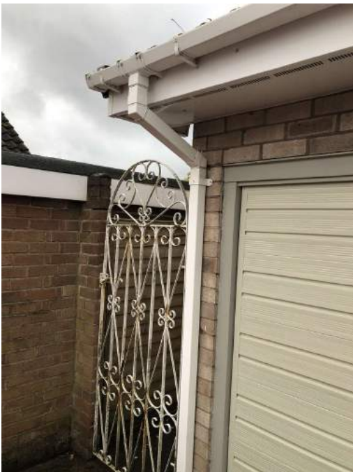
Gutter and downpipe.
