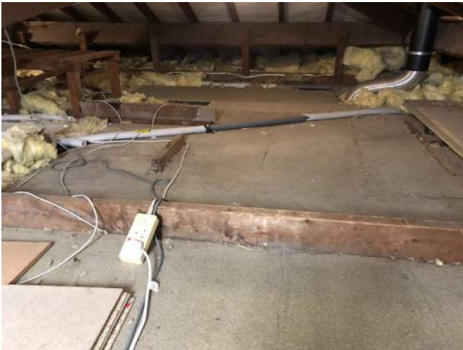
Roof space boarding.
