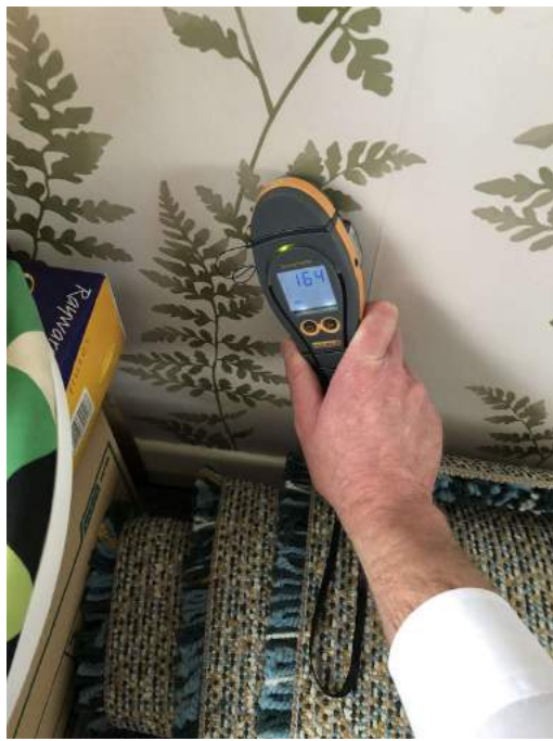
Internal wall damp check.
