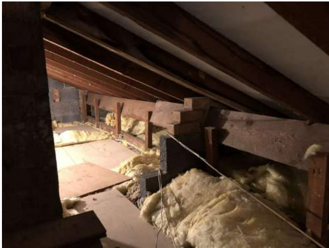
Purlin, hangers and rafters.
