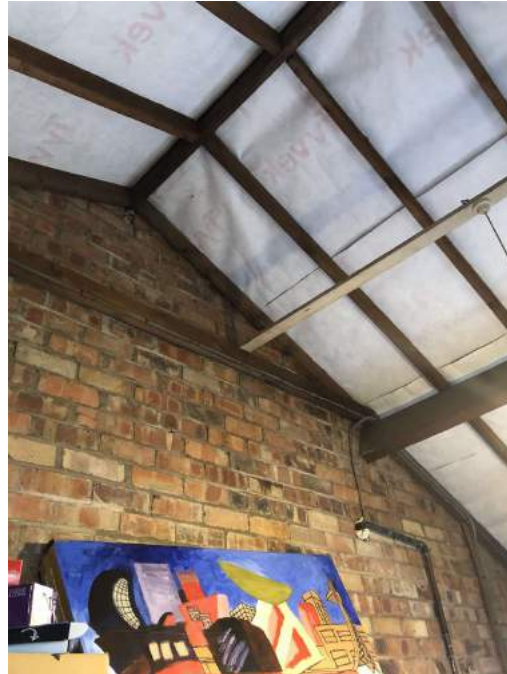
Garage roof structure.
