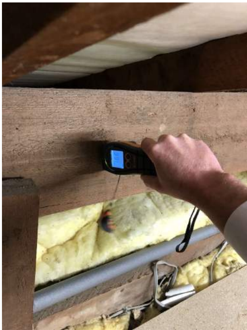
Purlin damp check.
